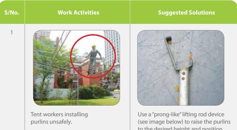
Use a "prong-like" lifting rod device (see image below) to raise the purlins to the desired height and position. In this way, workers can work from ground level when installing purlins.
