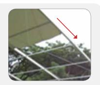
Some form of redesign may be required. One may consider installing the railings onto the tent frame members (see image below). The edges of the tent canopy are also required to be redesigned so that they can be slotted into the railings. In this way, workers are not required to work on top of tent structures.
