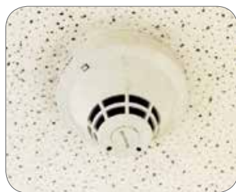
Figure 12: Ceiling-mounted smoke detector
