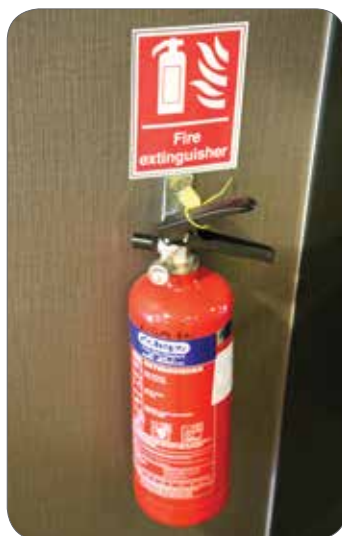
Figure 15: ABC dry chemical fire extinguisher
