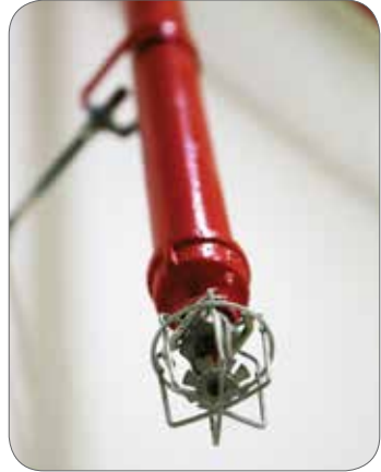
Figure 17: Standard sprinkler with guard
