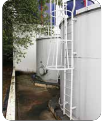
Figure 14: Example of a diked storage area
