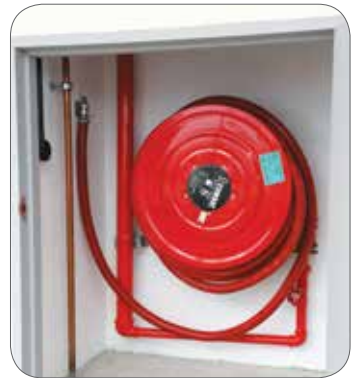
Figure 16: Fire hose reel located inside a cabinet
