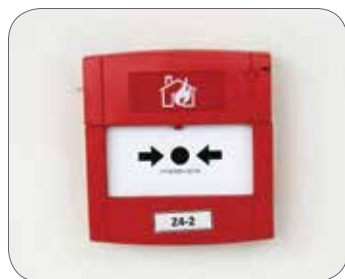
Figure 13: Fire Alarm Call Point
