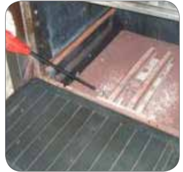
Figure 30: Lighting of pilot flame using a handheld spark generator
