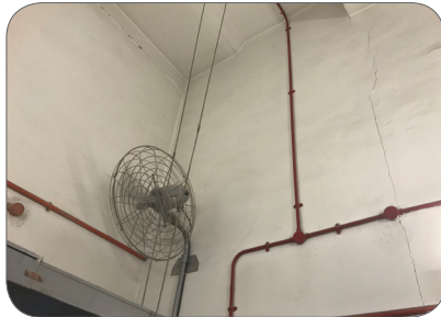
Figure 61: Cooling fan in motor room for workers may not be adequate
