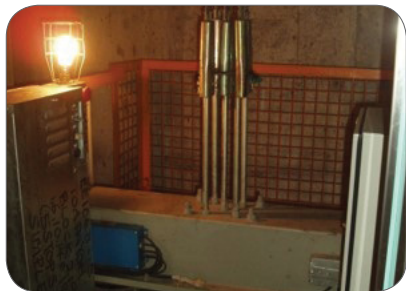
Figure 82: Adequate lighting with lamp guard, and car top barricade
