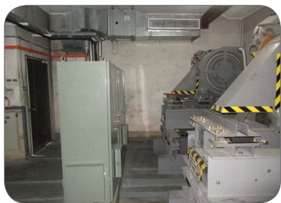
Figure 62: Example of an enclosed lift motor room designed and installed with ducted HVAC system
