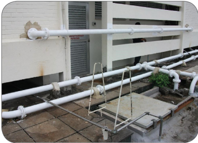
Figure 42: Motor room access with obstruction
