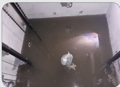
Figure 25: Flooded lift pit
