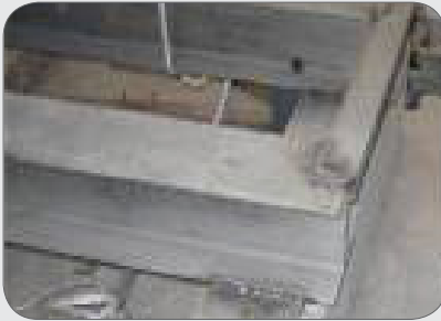
Figure 14: Sharp corner of metal beams
