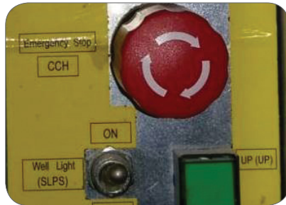
Figure 70: Emergency stop switch at lift motor room
