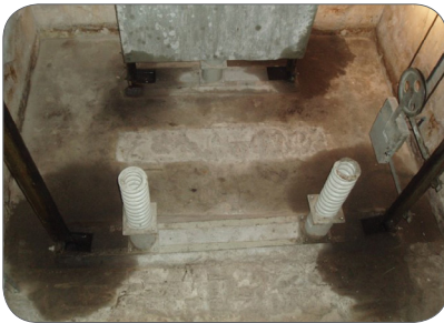
Figure 95: Clean & well lighted pit
