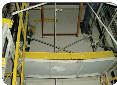
Figure 35: Falling off from improperly constructed platform
