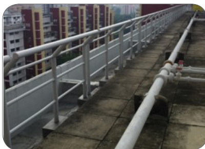
Figure 59: An example of roof top safety railing
