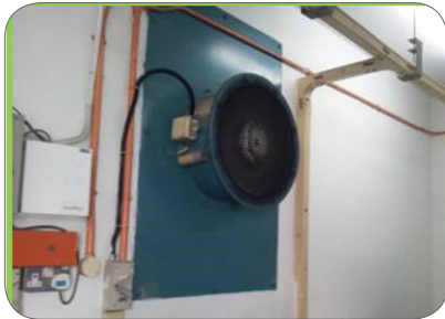
Figure 60: Exhaust fan with guarding providing cooling for machinery
