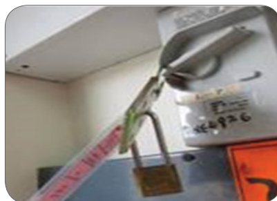
Figure 106: Example of lockout-and-tagout
