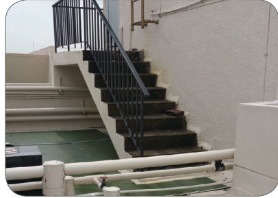
Figure 43: Motor room access with obstruction
