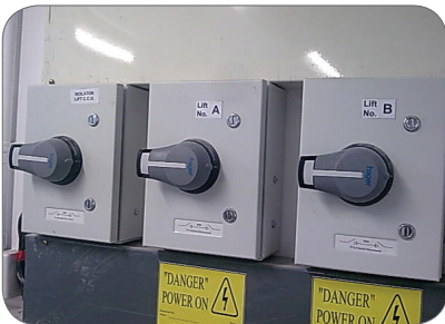
Figure 77: Examples of clear marking on lift isolators and distribution boards
