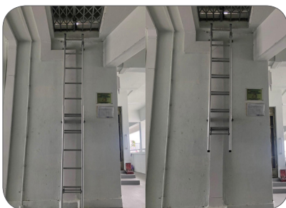
Figure 54: An example of vertical aluminium retractable cat ladder
