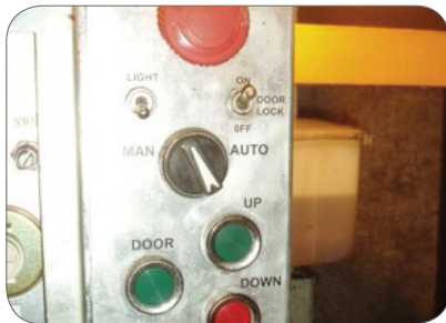
Figure 81: Operational switch set to maintenance
