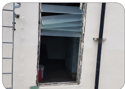
Figure 26: Electrical hazards due to rainwater entering lift motor room through damaged window panel
