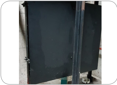
Figure 89: Counterweight screen installed in lift pit
