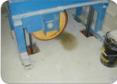
Figure 38: Objects falling through the openings in the machine room into the hoist way
