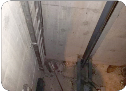
Figure 40: Vertical cat ladder to access to lift pits may be difficult and dangerous with the risk of falling
