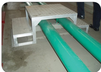
Figure 58: An example of access platform over pipes
