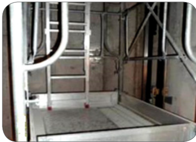
Figure 110: Use of scaffold in lift pit to reach the under carriage of the car lift
