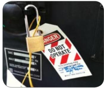
Figure 24: Example of a lock-out device.
