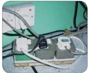
Figure 12: Haphazard electrical connections can lead to overloading and electrocution.
