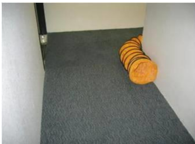
Figure 3: Renovation fumes from a room being exhausted into the common corridor.
