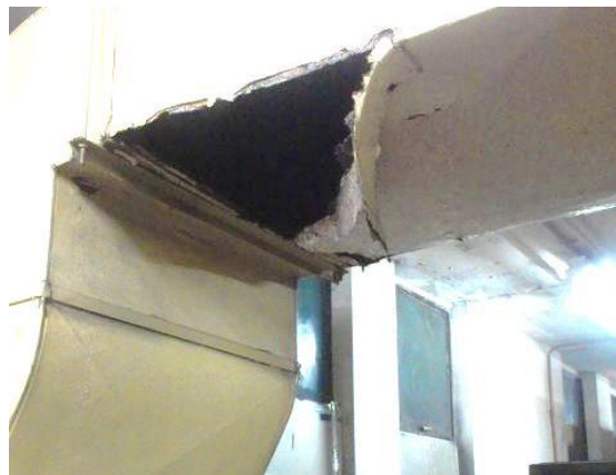
Figure D2: Damaged outdoor air intake ducts may allow PM to bypass the filtration system and infiltrate the building.
