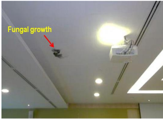
Figure 4: Fungal growth on ceiling board.
