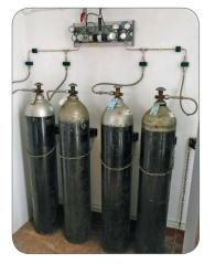
Figure 13: Gas cylinders secured in an upright position and stored in a cool, well-ventilated area.
