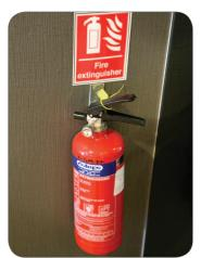
Figure 30: ABC dry chemical fire extinguisher.
