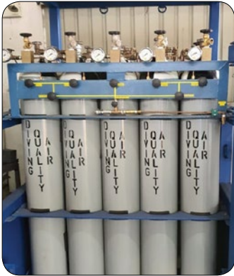
Figure 9: HP cylinders in quads.
