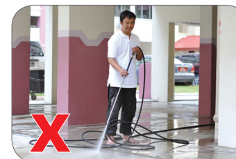
Figure 15: Spray jet (unsafe use) • Lack of helmet, gloves & boots • Lack of warning sign and tape • Hose tangled around feet
