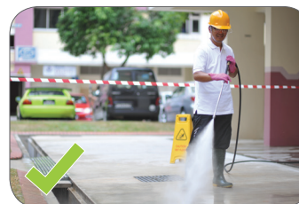
Figure 14: Spray jet (safe use) • Wear non-slip rubber boots and impervious gloves • Wear safety goggles and ear plugs
