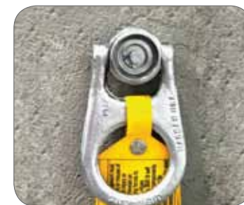
Figure 2: Example of a cast-in eyebolt anchor.
