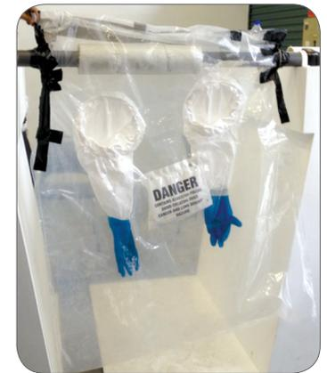
Figure 15: Glove bag containing asbestos waste.
