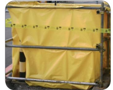
Figure 9: Example of a self-supporting temporary enclosure.
