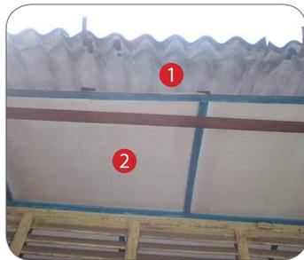
Figure 2: Asbestos used in building roof sheets and ceiling boards.
