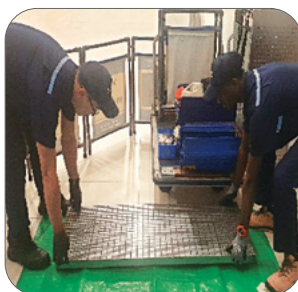
Figure 20: Risk of finger cut/laceration when load drops.
