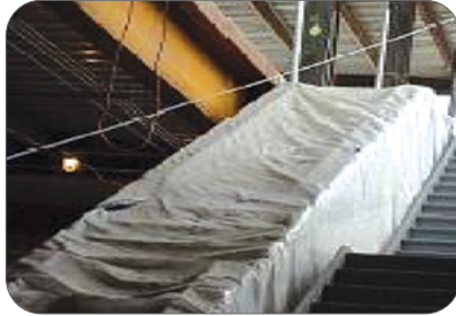
Figure 37: Wire rope lifeline used for fall protection.
