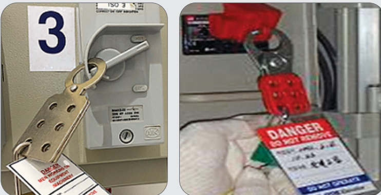
Figure 27: LOTO for the main-line switch of Esc/MW.
