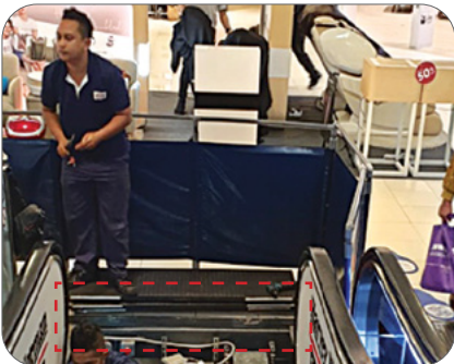
Figure 24: Limited working area beyond escalator pit.
