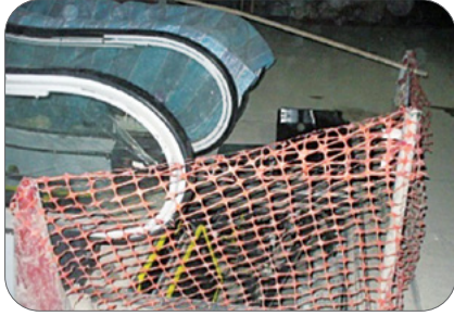
Figure 10: Fall into escalator opening during installation.
