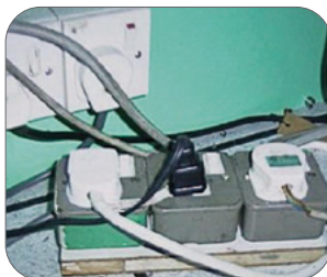
Figure 7: Overloaded circuits and plugs.
