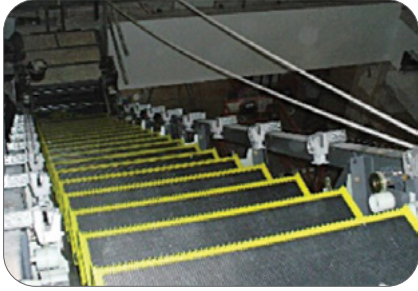
Figure 9: Fall off from open sides of escalator truss.
