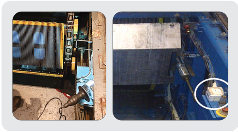
Figure 31: Provision of additional socket for portable light.
