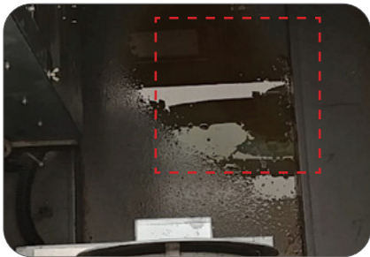
Figure 15: Oil spillage on floor surface in escalator motor room.
