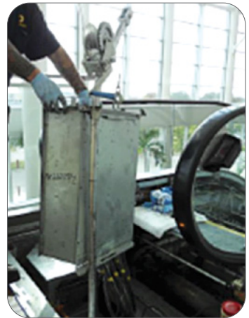
Figure 35: Controller lifting tool.
