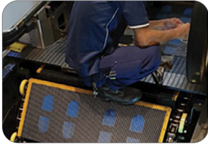
Figure 12: Fall into escalator opening during servicing.
