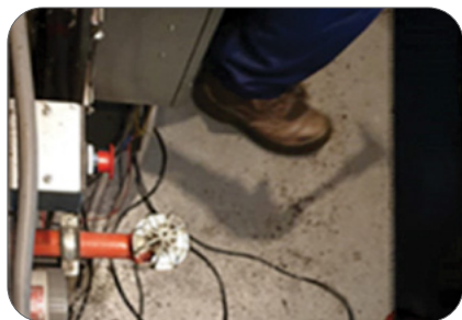
Figure 17: Tripping on loose cables and sprinkler pipe at escalator machine room/pit.
