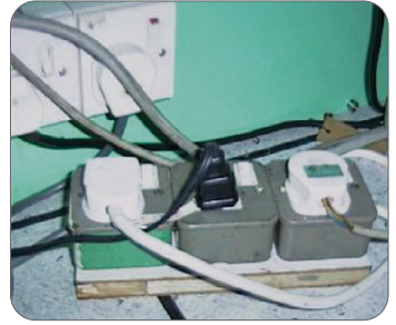
Figure 18: Haphazard electrical connections can lead to overloading and electrocution.
