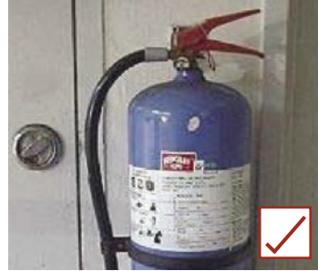
Place fire extinguishers near flammables
