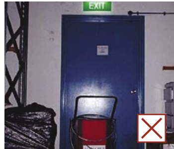
Do not obstruct fire escape passages
