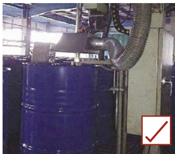
Use a local exhaust ventilation during chemical filling
