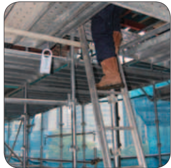
Figure 18: Safety shoes and boots provide limited protection for the feet from light falling objects.
