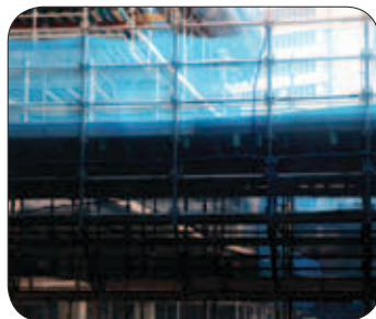
Figure 9: Toe-boards prevent items from falling off the surface of the platform of the scaffold.
