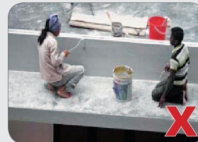
Workers painting near open edge of roof without any fall restraint or arresting systems.
