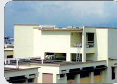
Flat non-fragile roof with low parapet walls.
