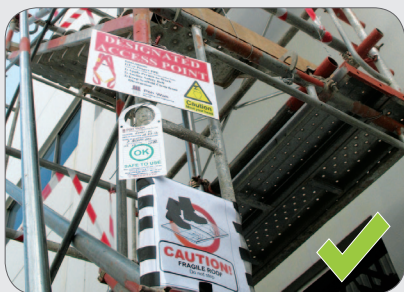
Fragile roof surfaces are identified and warning signage is provided at designated access point(s) onto roof.
