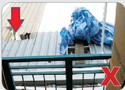
Fragile roof surface is not identified before work and no safety signage is used to warn workers of hazard.
