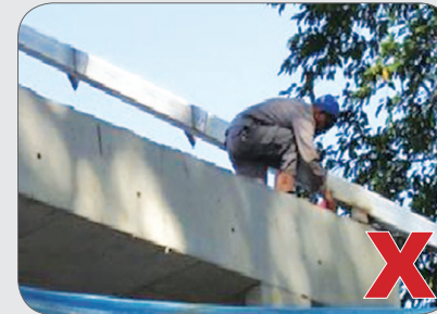
Working on roof without any edge barricade.
