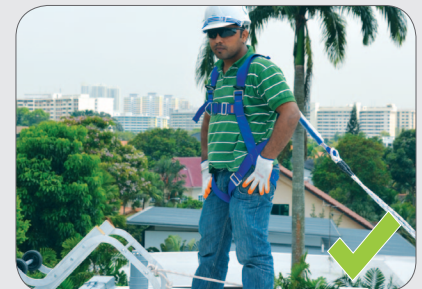
Fall restraint systems used to prevent workers from moving close to edge of roof.
