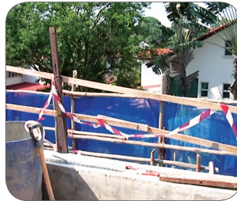
Figure 10: Examples of ineffective barricades.
