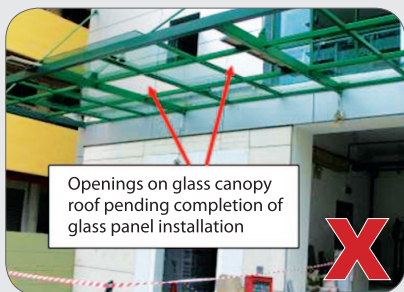
Installation of glass canopy roof without proper access and measures against falling through roof openings.
