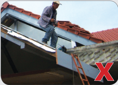
Roof access ladder is not secured to structure at bottom and top rungs.
