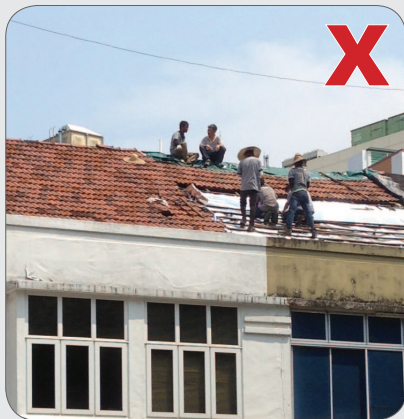
Workers on roof without safety harness and anchorage.
