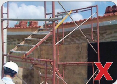
Unsafe scaffold used to access roof.
