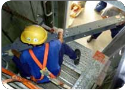
Figure 43: Manual handling within the confines of the shaft can be difficult.
