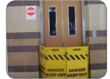
Figure 57: An example of using lift barrier to prevent unauthorised access.
