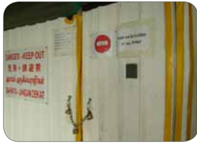
Figure 56: Example of hoarding during lift modernisation.
