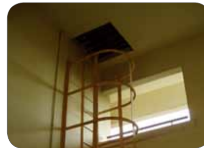
Figure 47: Example of cat ladder with ringed hoops.
