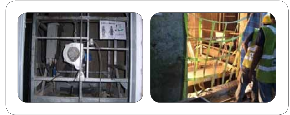
Figure 26: Falling off suspended or moving platforms such as gondola (left) and false cars (right).
