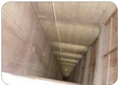
Figure 36: Wooden partition used to isolate hoist way to prevent workers from being hit by items accidentally dropped from other hoistways.
