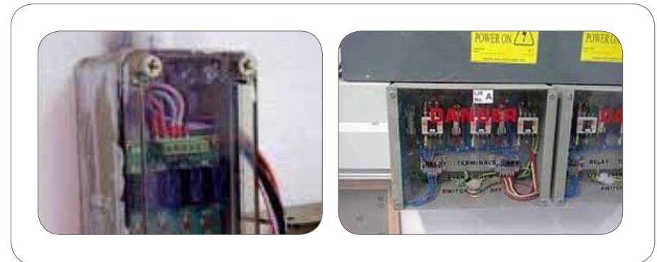
Figure 50: Examples of finger-safe terminal block.
