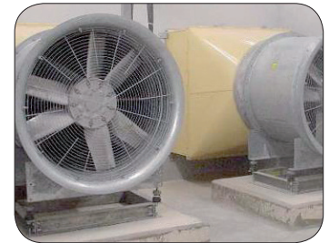
Figure 15: Example of local exhaust ventilation.
