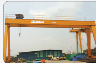
Example of a Gantry Crane
