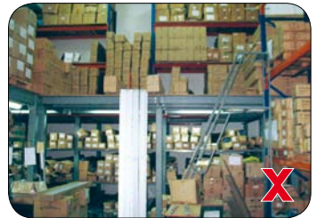
Mezzanine floors with no barricades.
