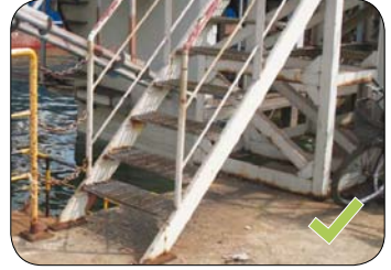
Stairs are fitted with handrails.
