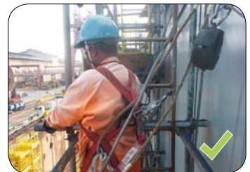
Safety harnesses have to be worn properly and they have to be securely anchored.
