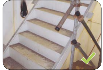
Handrails at open edges of stairway.
