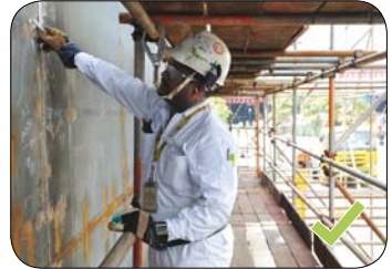
Working platform with guardrails and toeboards installed.
