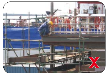
The worker is working on an unguarded side without a working platform. He is also not wearing a safety harness.
