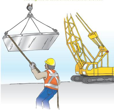
Use tagline with sufficient length and diameter so that the tagline can be easily gripped and the load stabilised.
