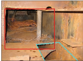
Steel removal work done on top side tank.
