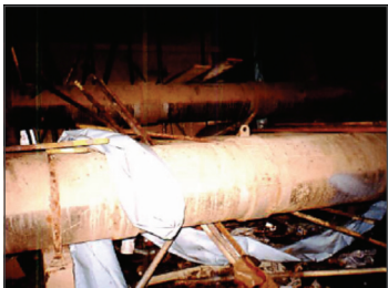
The scaffold tubes struck a structure and fell while they were being winched up.
