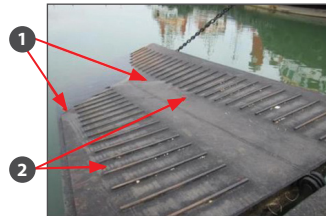
Photograph showing the pair of slanting tyre marks and the skid marks over the edge of the ramp.
