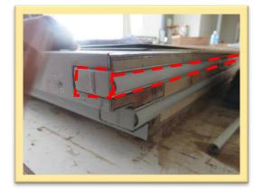
Pic 3: To cut the groove (highlighted in red) for installing bottom panel of timber door frames.
