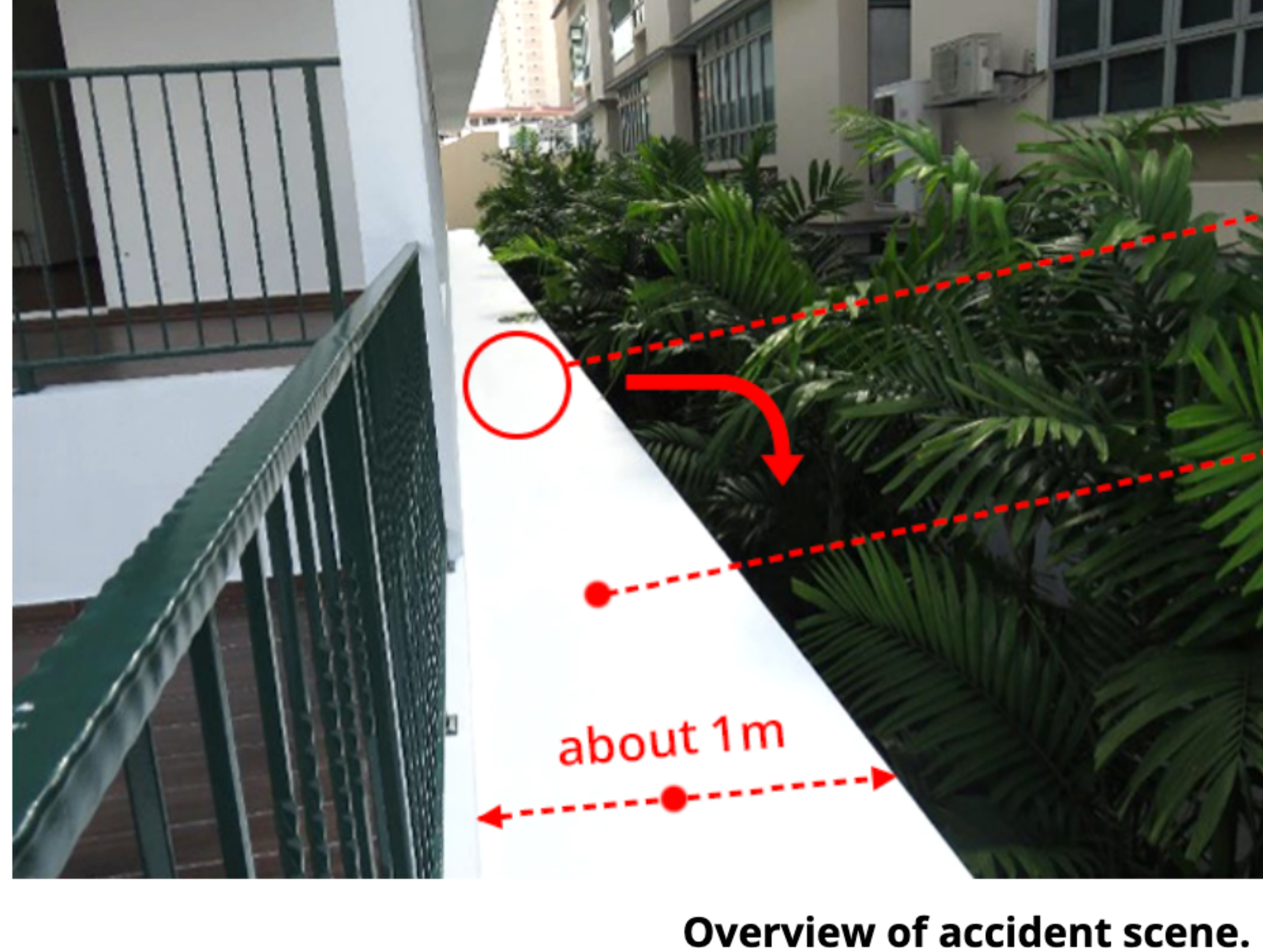
Overview of accident scene.
