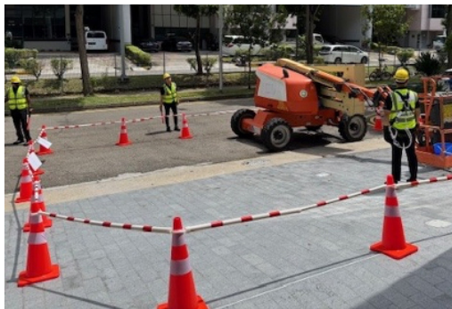
Work area cordoned off.
