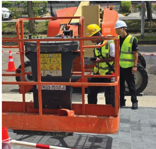
Carrying out pre-use MEWP inspection.
