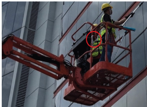
Worker with both feet on the platform of the MEWP.
