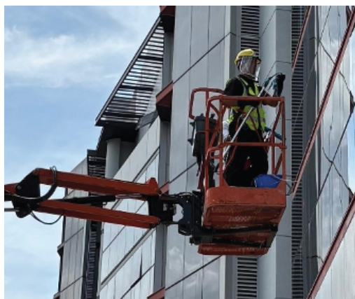
Worker with both feet on the platform of the MEWP.
