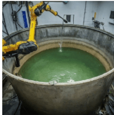
Tank is filled with water and drained to remove residual chemicals before entry
