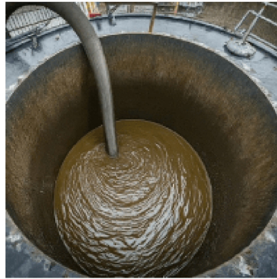
Decomposing sludge is removed using a pump
