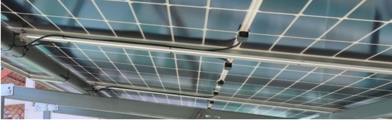
Figure 3: Example of cables secured under a solar panel.
