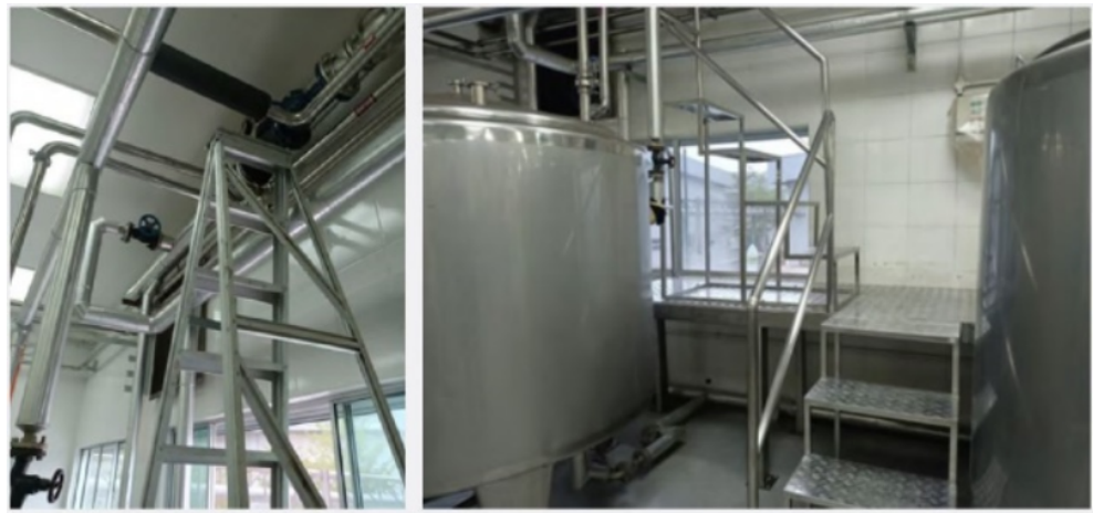
Before: Operator used a ladder to access the steam valve
