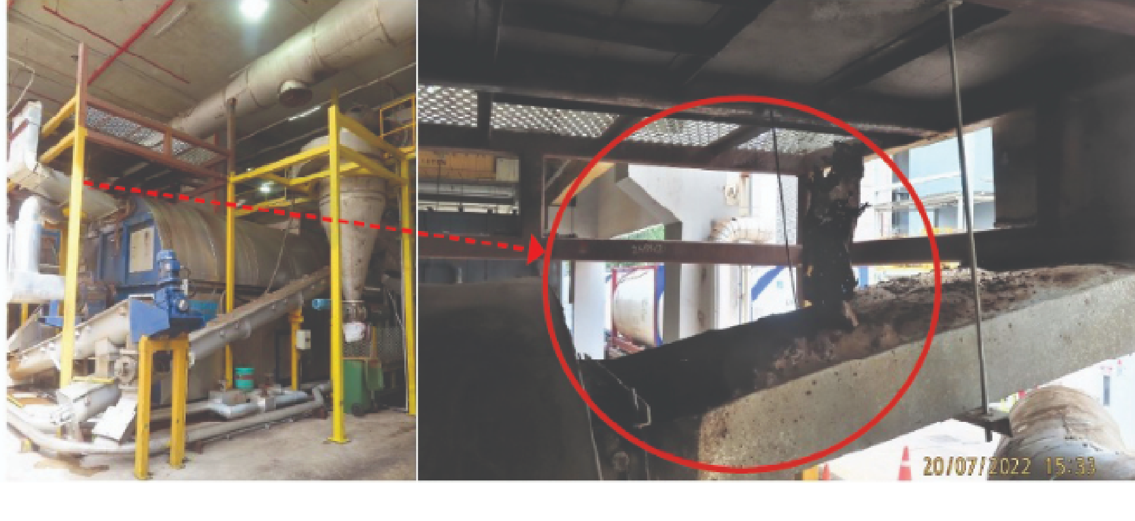
Figure 3: The force from the dust explosion spread to the relief vent which blasted open.
