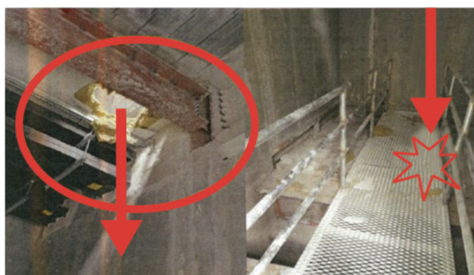
Figure 2: The boarding through which worker fell (left image) and the metal walkway where the worker landed (right image).
