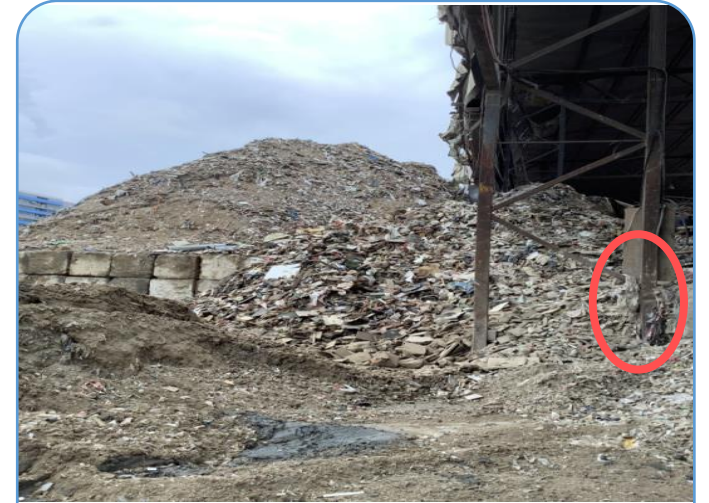
Storing Material against Load- bearing Structures
