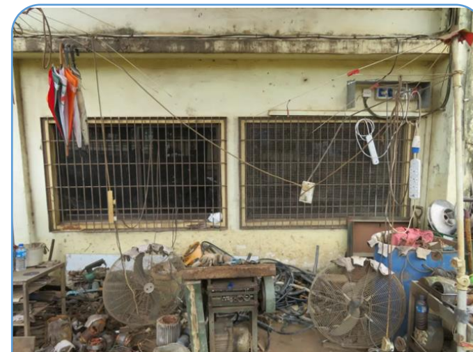
Usage of Non Weatherproof Socket and Extension Socket
