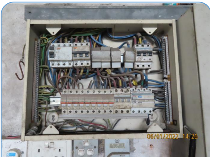
Exposed Live Conductors in Distribution Box (DB)
