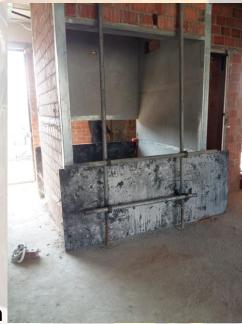
Simple timber bariicade with GI pipes in place at lift pit to prevent falls
