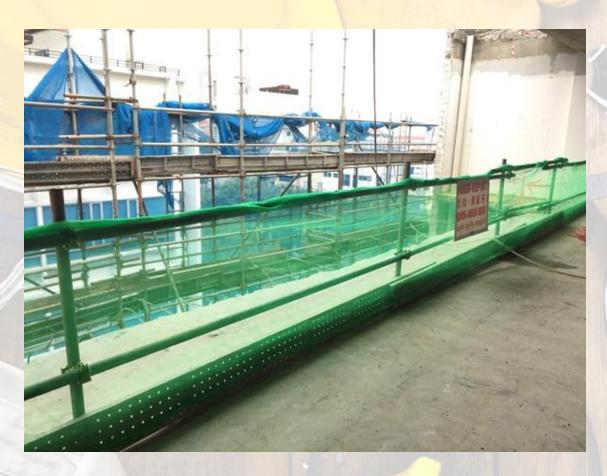
Safety barricades with toe-board and safety netting installed at open sides.
