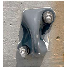
Safe Arrest System and Anchorage Points
