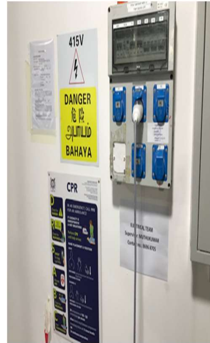
Temporary DB with Warning Sign, Poster on CPR and Permit-to-Work
