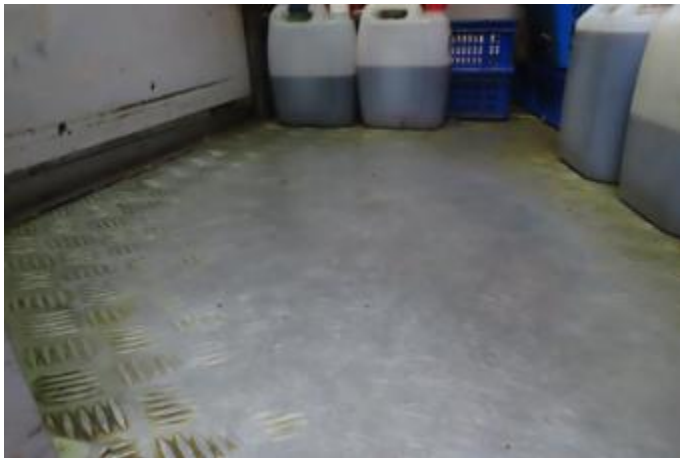
Slip resistant treads worn out
