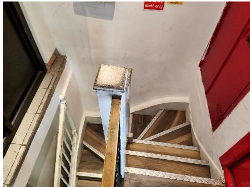
Staircase leading to the basement
