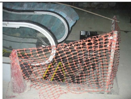
Figure 10: Fall into escalator opening during installation
