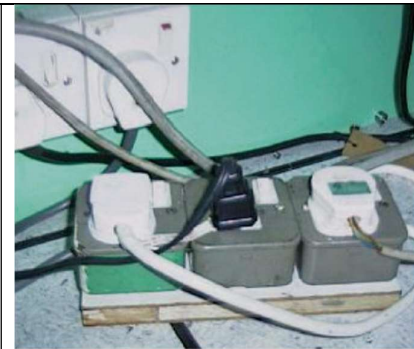
Figure 7: Overload circuits and plugs
