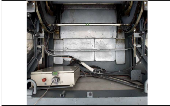
Figure 32: Good housekeeping for the pit
