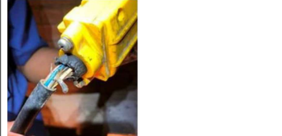
Figure 6 : Damaged electrical cords
