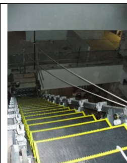
Figure 9: Fall off from open sides of escalator truss
