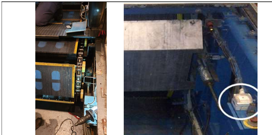
Figure 31: Provision of additional socket for portable light
