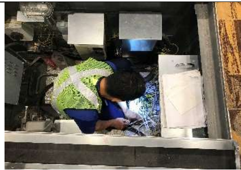
Figure 8: Electrical shock when contact with live electrical panel/ cables.
