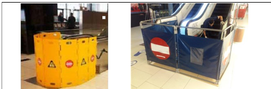
Figure 26: Barricade to prevent unauthorized entry
