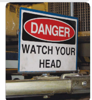
Figure 16: Erect warning signs for low overhead structures such as pipes.
