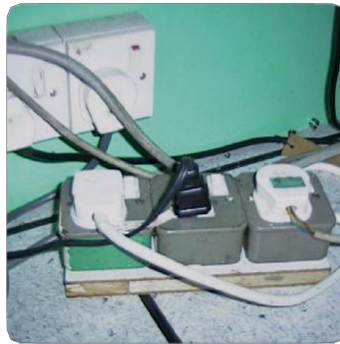
Figure 18: Haphazard electrical connections can lead to overloading
