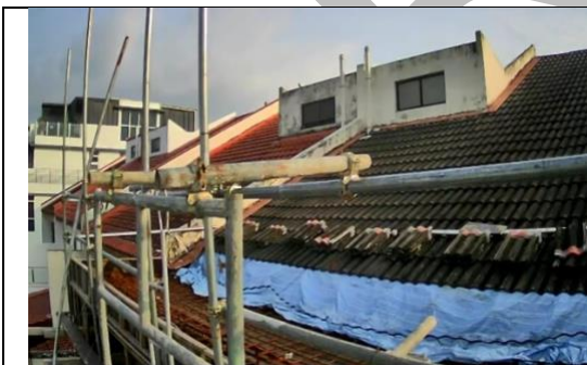
Figure 5: Working at height activity
