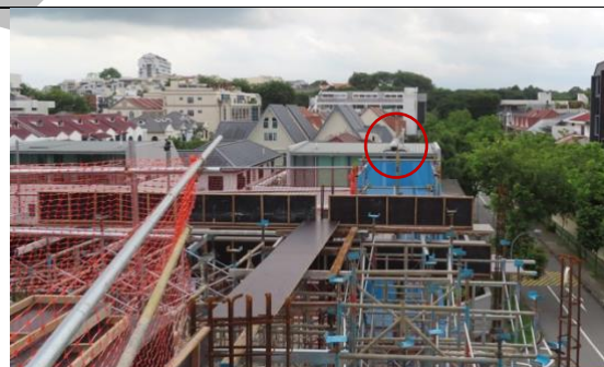
Figure 6: Working near the construction of support structure
