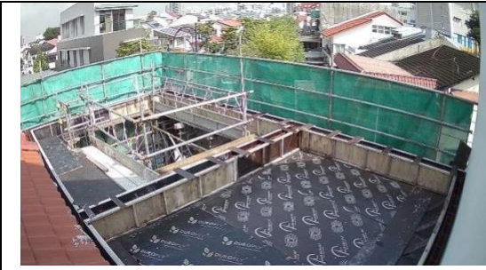
Figure 7: At a floor of a building under construction
