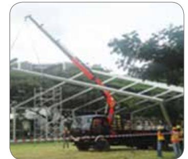
Figure 8: Lifting of tent structure using lorry crane.
