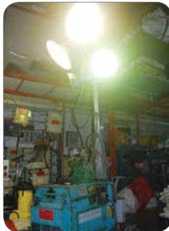
Figure 5: Example of a lighting tower.
