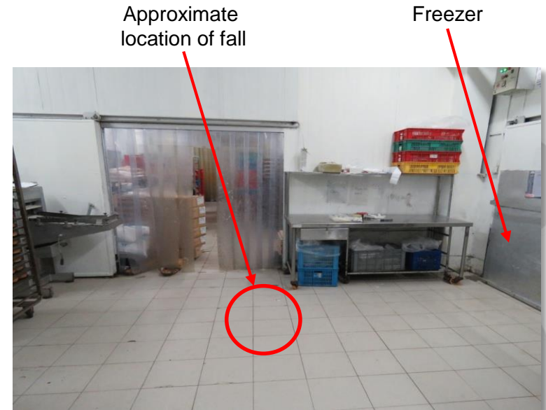
Figure 5: Scene of the accident where the worker slipped and fell.
