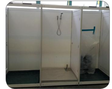
Figure 13: A decontamination facility consisting of three separate compartments (clean, shower and dirty areas).
