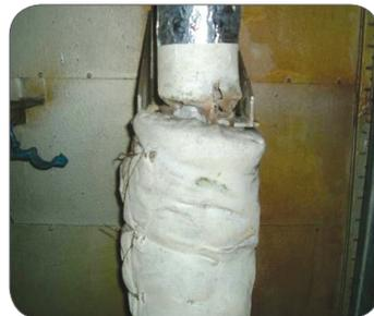
Figure 3: Asbestos cloth wrapping with asbestos lagging of exhaust pipe.
