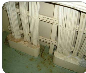
Figure 4: Asbestos-containing cable penetrations used on ships.
