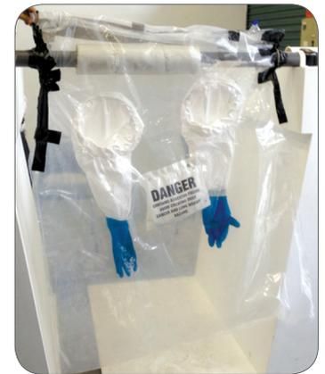
Figure 15: Glove bag containing asbestos waste.
