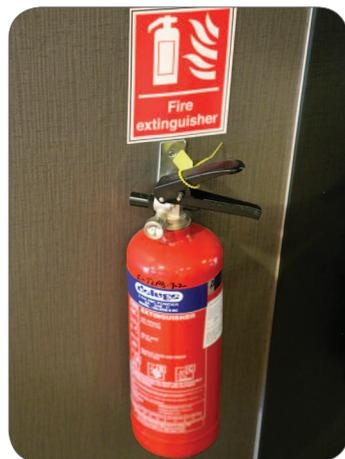
Figure 30: ABC dry chemical fire extinguisher.
