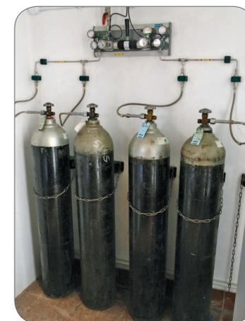
Figure 13: Gas cylinders secured in an upright position and stored in a cool, well-ventilated area.
