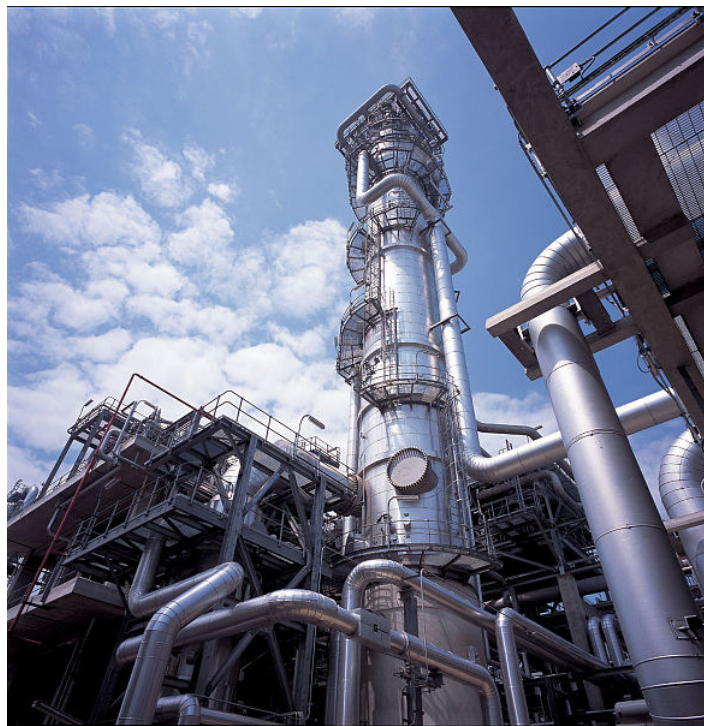
Figure 4: A typical column in a chemical plant
