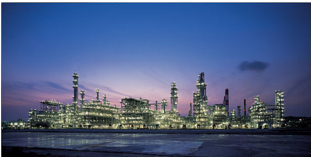
Figure 1: A typical oil refinery
