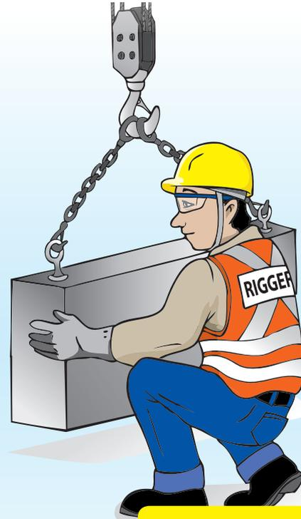
Make sure the load is stable, balanced and secured before any lifting operation.
