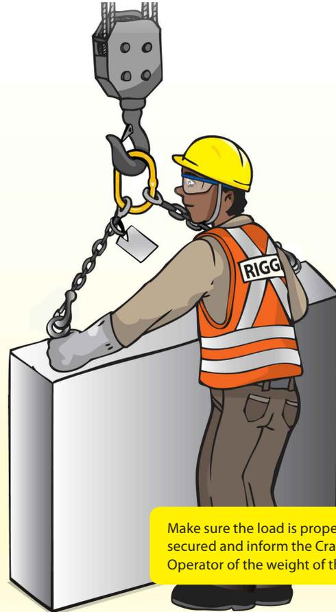
Make sure the load is properly secured and inform the Crane Operator of the weight of the load.
