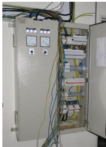
Figure 1: The electrical distribution board that the worker was dismantling.
