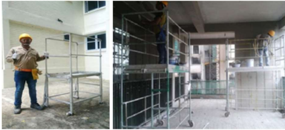
Figures 2 and 3: Examples of access platform. Image source: Courtesy of TEAMBUILD
