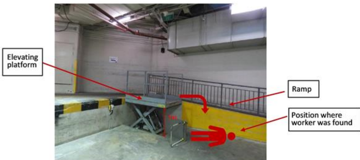
Overview of accident scene.
