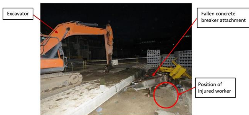
Overview of the accident scene.
