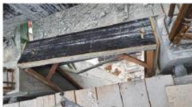
Structure used to bridge the gap.
