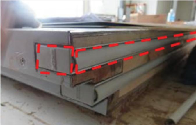
*To cut the groove (highlighted in red) for installing bottom panel of timber door frames*
